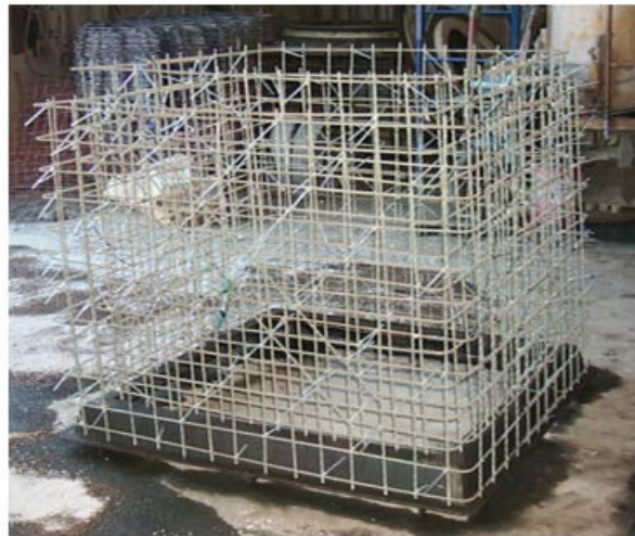
Figure 2: A Complete GFRP cage before concrete casting
