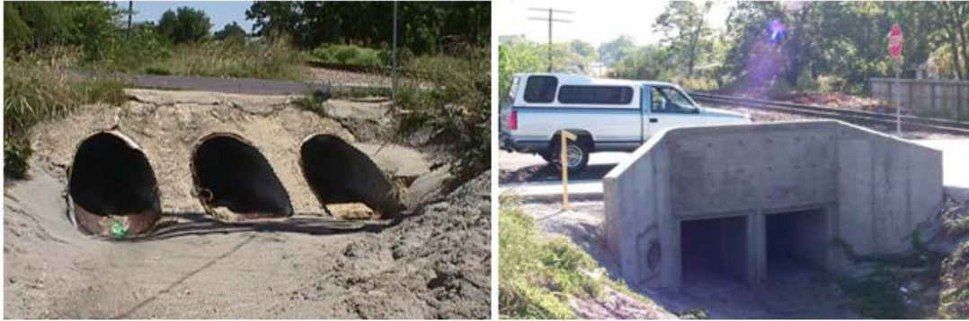
Figure 1: Old (left) and new (right) Walker Bridge
