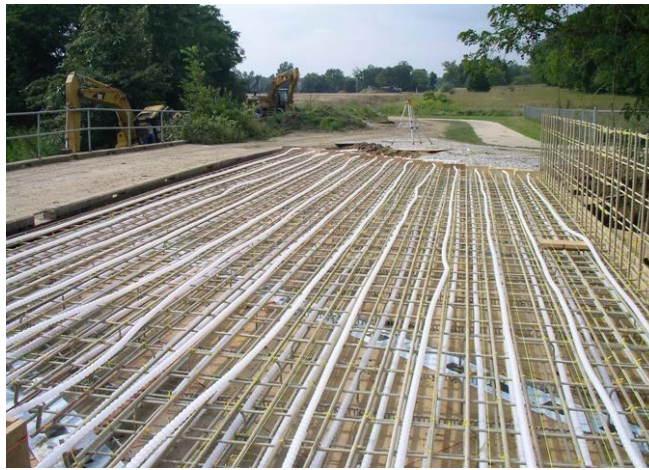
Figure 4: Southview Bridge Deck Top-GFRP Layer and CFRP Tendons
