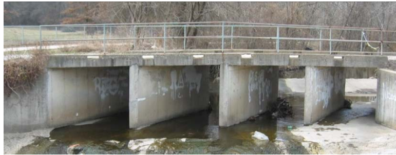
Figure 3: A View of the Former Southview Bridge
