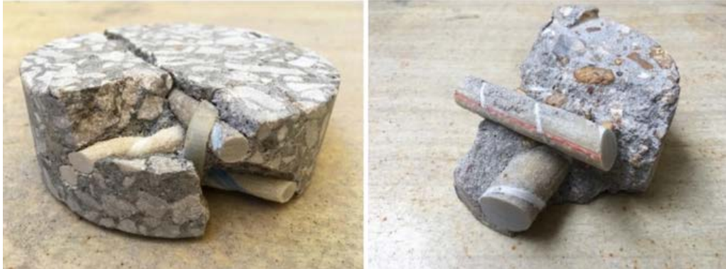
Figure 5: GFRP coupons extracted from the concrete cores of Walker (left) and Southview (left) Bridge
